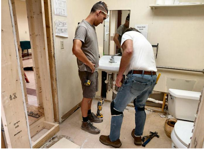
A Whitecap carpenter and a plumber prepare to upgrade a bathroom.
